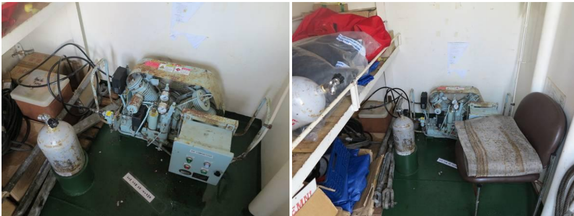
Figure 8.14 – Type of B.A. compressor
