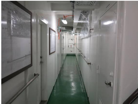
Figure 7.8– Repaired Captain’s deck
