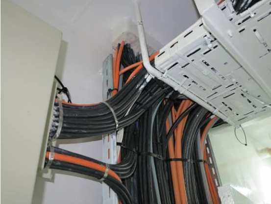
Figure 7.5– Repaired cabling in Captain’s deck
