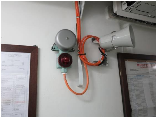
Figure 7.7– Repaired fittings in Captain’s deck
