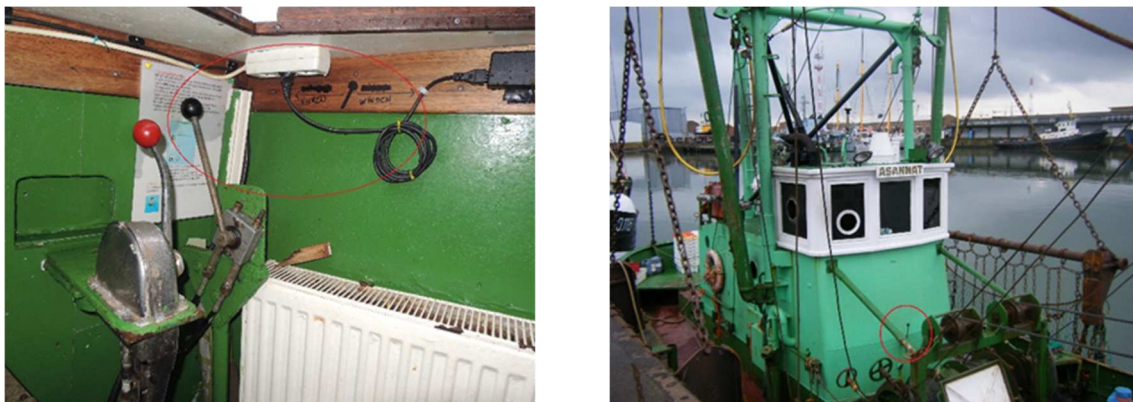
Figure 17 - winch control valves inside the wheel house and on facing of superstructure of fv Z582 ASSANAT (archive pictures)
