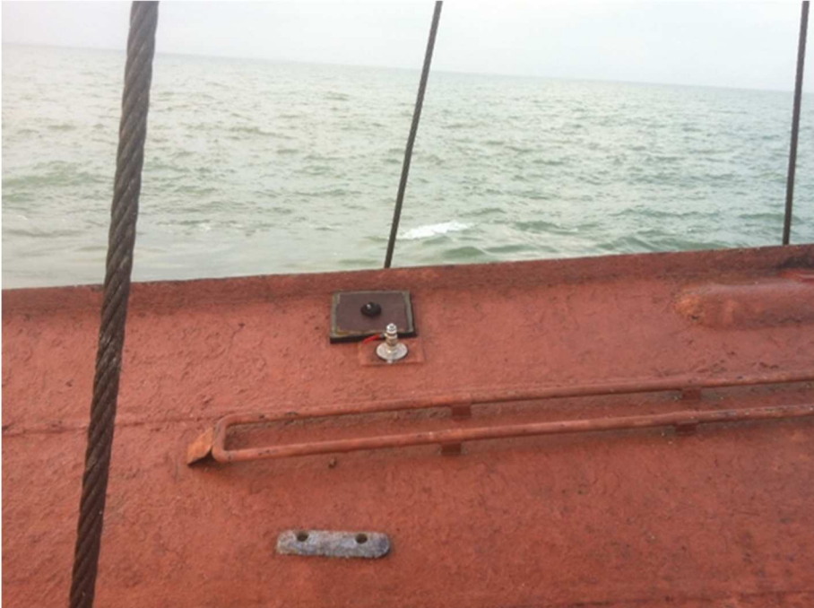
Figure 5 - Hot taps placed onto hull of Z582 ASSANAT
